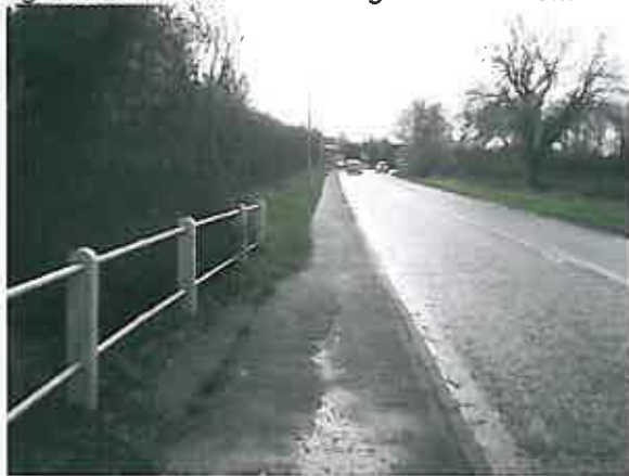
Figure 3.4: Welford Road – bridge across stream
