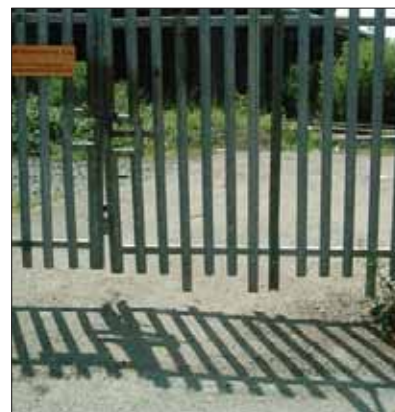
Galvanised railway fence
