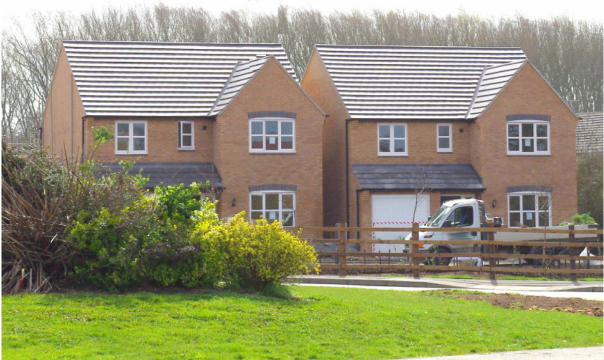
Dwellings nearing completion at Pipistrelle Way, Oadby.
