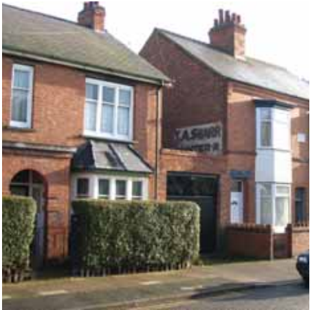
Northeast end of Fairfield Street
