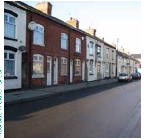
West side of Station Street
