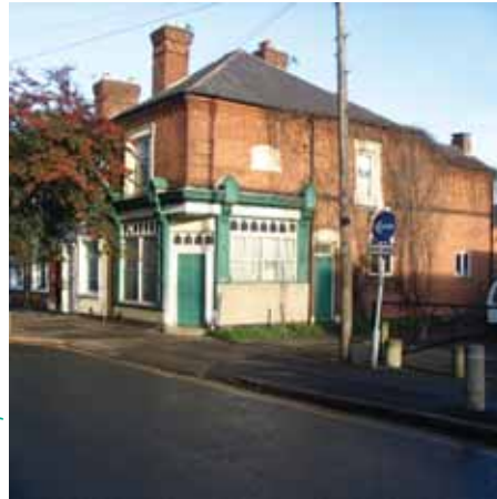
C19 shopfront on east side of Glen Gate
