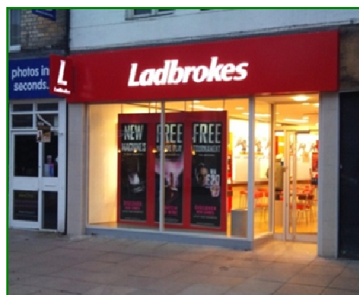
Shutters behind the glass frontage can reduce detrimental impact and contribute to retained historic interest and the integrity of the original frontage (Stockport)
