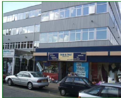
Poor quality architecture and floor plates not attractive to modern retail
