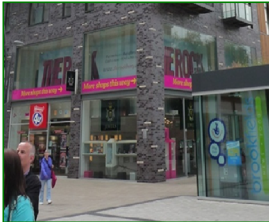
Modern shop front design with double height frontage appropriate for new development (Bury)
