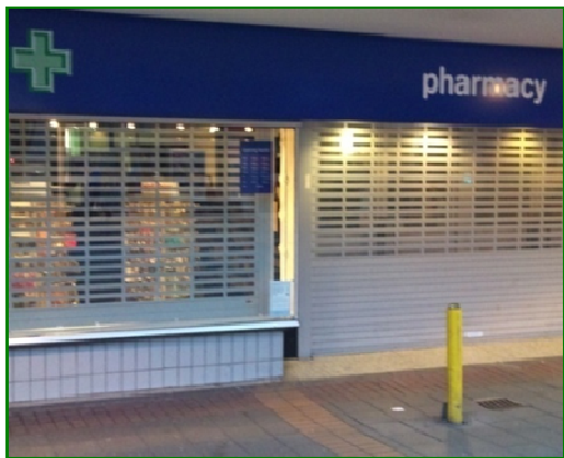
An example of perforated shutters enabling views into the shop but maintaining security (Sale)
