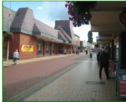
Blank / impermeable frontage along Bell Street
