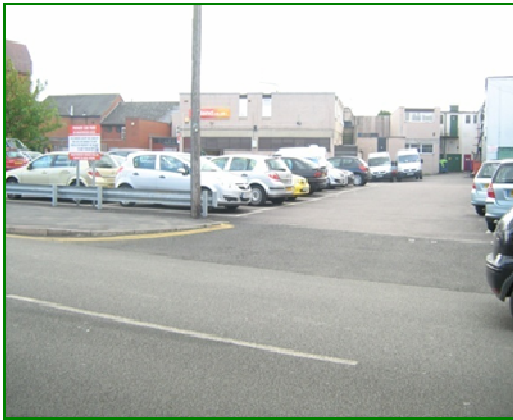
Car parking and rear servicing creating an unwelcoming first impression
