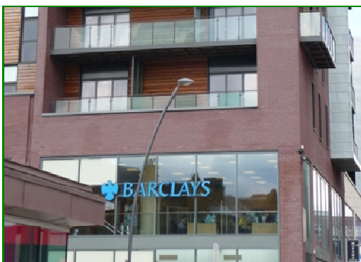
Residential development above ground floor retail / commercial use (Bury)
