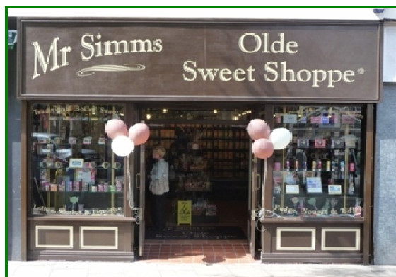
Traditional shop front design reflecting occupier. A good example of independent retail (Bury)
