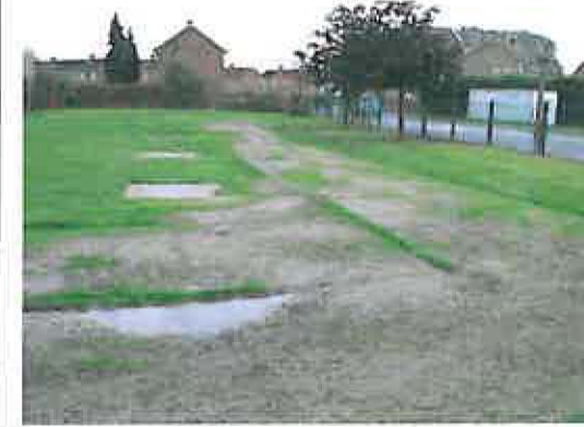
Poor drainage and pitch quality in need of repair at southern end of site
