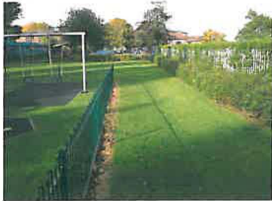
Poorly assimilated play area with duplicated fencing in need of enhancement to improve appeal and use
