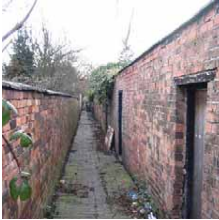
Passageway to the rear of the cottages
