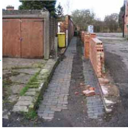
Path and wall to the pub carpark
