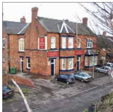
Public house (former Railway hotel)
