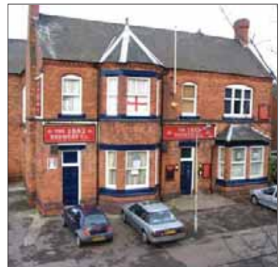
Public house (former Railway hotel)
