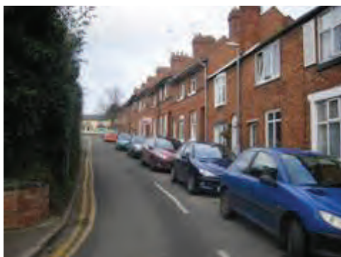
Albion Street Terrace Housing
