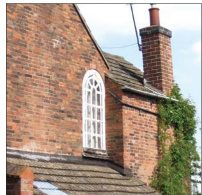
2 Newgate End - gable window
