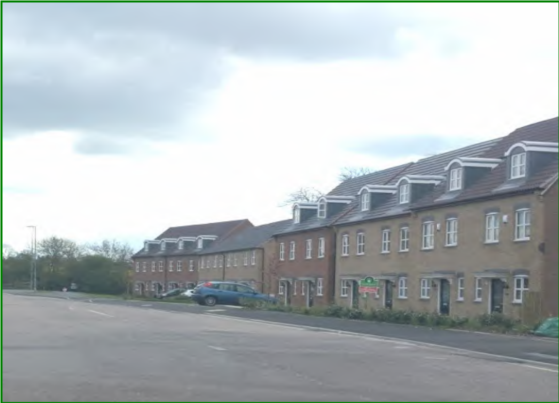
Completed affordable units at Pipistrelle Way, Oadby
