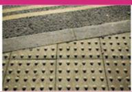
Dropped kerbs facilitate non stepped access, usually between the footway and carriageway. These should be accompanied by tactile paving, which provides a distinctive, raised surface profile to be detected by both sighted and visually impaired users.
