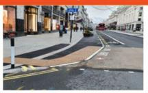
A section of footway extended out into the carriageway to reduce the crossing distance and improve visibility for pedestrians. It is also intended to limit the speed of vehicles.
